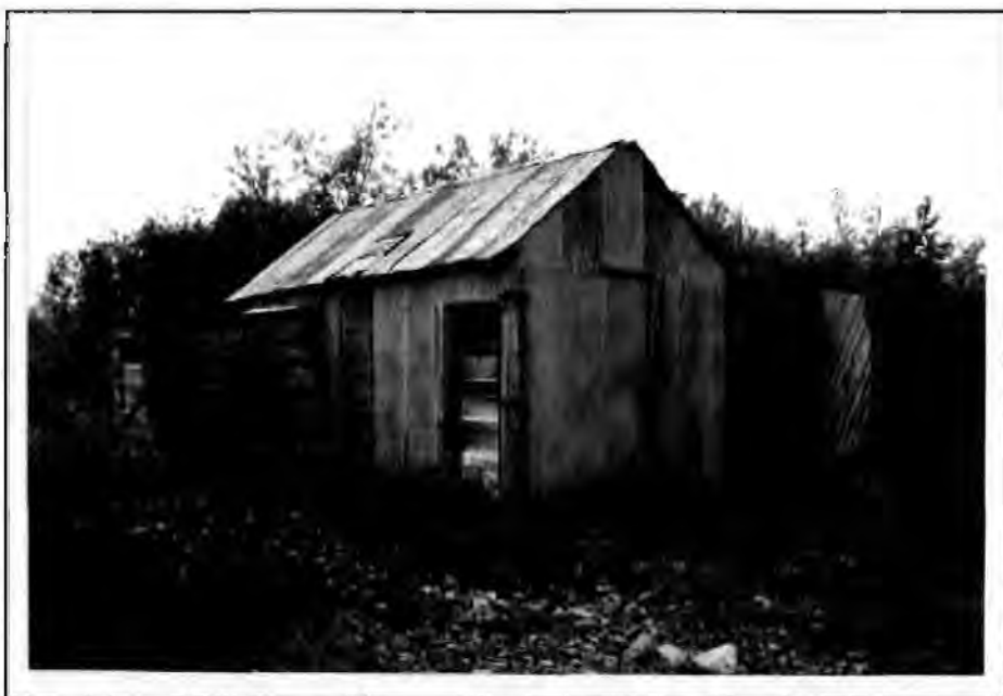
Figure 57. The Matheson Garage, 1993. The view is looking southwest.
